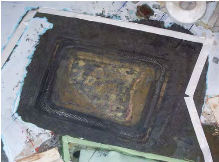
Scarf repair area
